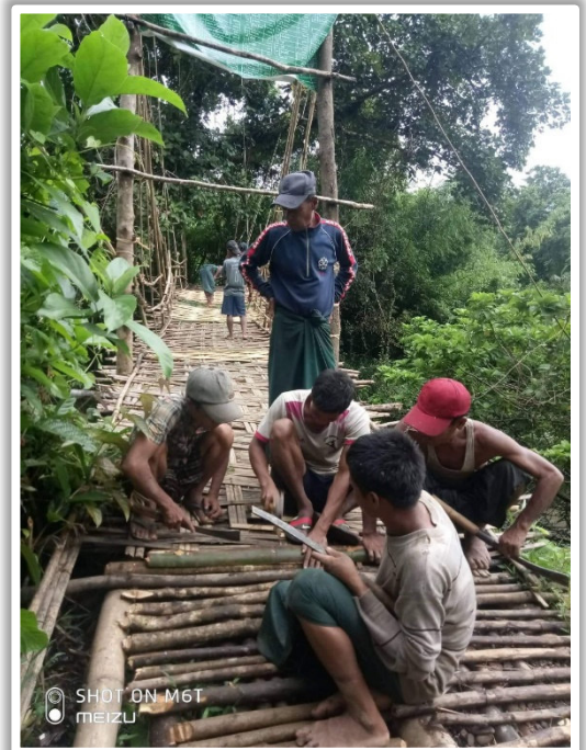
Repairing a bridge in Pyin Taung (Rakhine)
